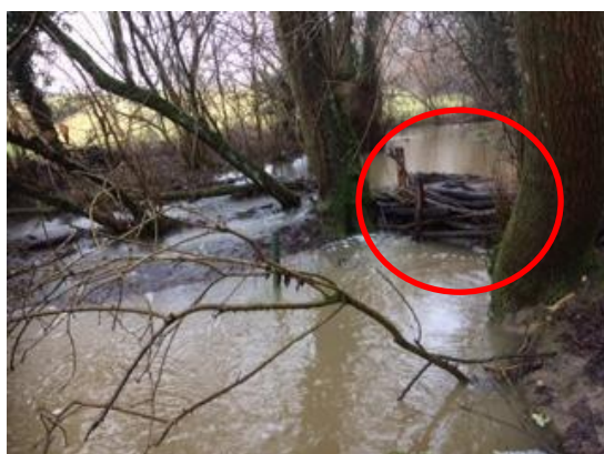
Fig. 2 Debris dam constructed in Lag Wood (winter 2016) and simple cross design for debris dams, shown by University of Brighton to be as effective.
