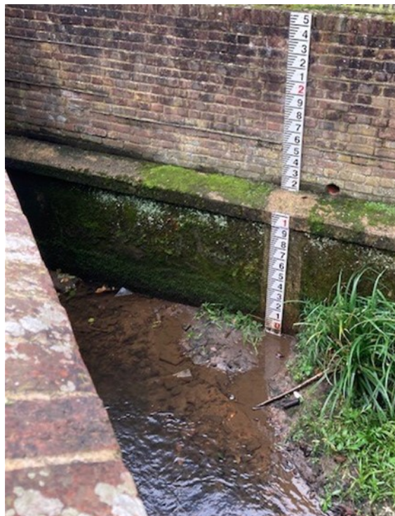
Water Level Gauge Board at Spitalford Bridge
