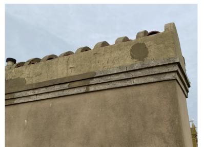
Cracked render to the top of the chimney stack.
