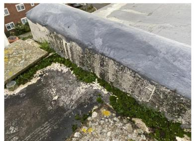
Cracking to the rendered party wall on the south side of the four-storey projection roof.
