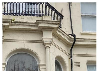
Deteriorated paint finishes to the front elevation wastepipe.
