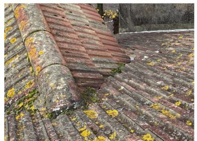
Poor quality narrow roof valleys either side of the front dormer.
