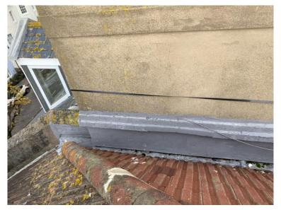
Valley between north pitch and the chimney stack, believed to be leaking into the top floor flat. Attempts have been made to prolong the life of this valley by coating it with a liquid system.
