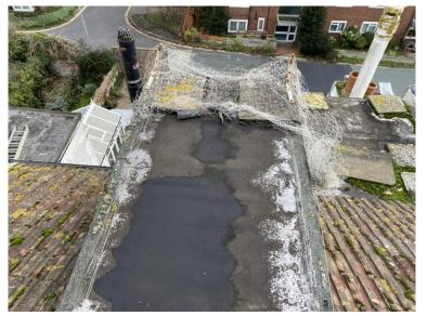
Heavily worn felt over the rear dormer flat roof.
