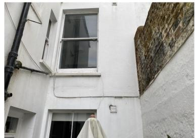
Cracked render to the rear elevations.
