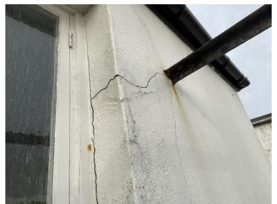
Cracked render and masonry to the rear of the four-storey projection.
