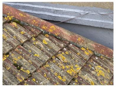
Deteriorated mortar bedding to the roof hip and ridge tiles.
