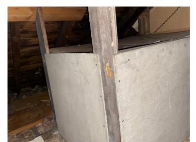
Presumed asbestos fibre cement board to the cold-water tank in the roof space.
