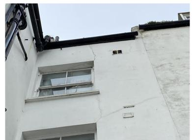
Cracked render to the rear elevations.
