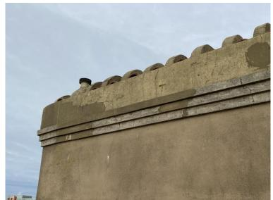
Cracked render to the top of the chimney stack.
