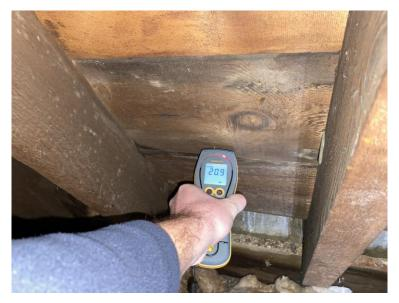
Elevated moisture readings and some mould to the timber rafters and close boarding in the roof space above the top floor flat.
