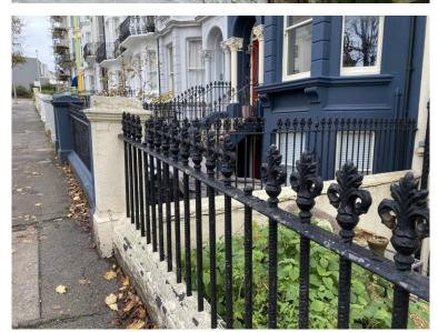
Flaking paintwork and minor corrosion to front garden railings.
