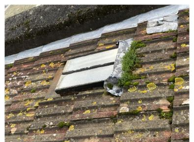
Corroded and rotten frame to the rear roof light with vegetation blocking the perimeter gutter channels and flashings.
