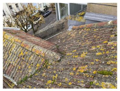
Poor quality valleys either side of the front dormer gable roof where it meets the front roof pitch.
