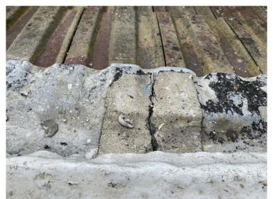
Split lead cover flashing to the front dormer.
