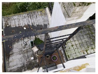
Advanced corrosion to the rear roof fire escape ladder.
