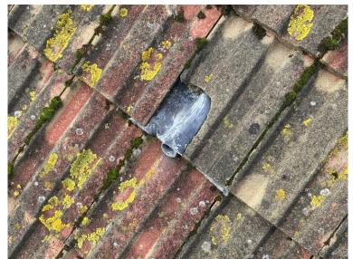
Broken roof tile to the rear pitch and cold-water tank overflow pipe.
