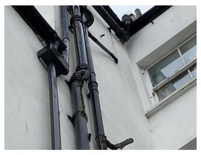
Deteriorated rear uPVC downpipes and cracked and leaking cast-iron soil and vent pipe.
