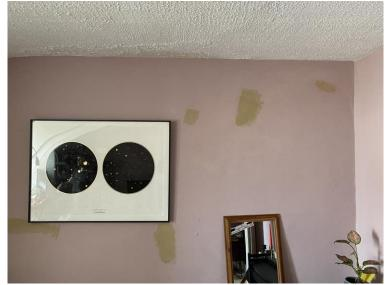
Water damaged and poorly patch repaired north wall to the top floor flat living room.
