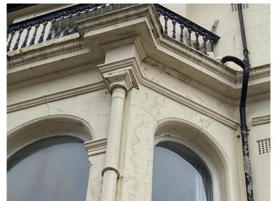
Cracked render to the front elevation bay window.
