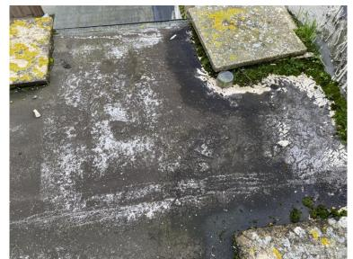
Heavily worn felt over the four-storey projection roof.
