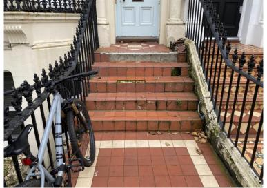
Damaged and missing quarry tiles to the entrance steps.
