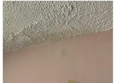
Water stained and saturated ceiling adjacent to the north wall of the top floor flat's living room.
