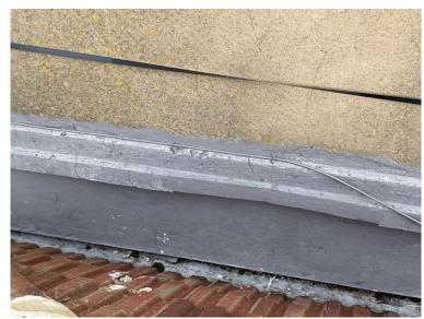
Cracked low level render to the chimney stack coated with a liquid system.
