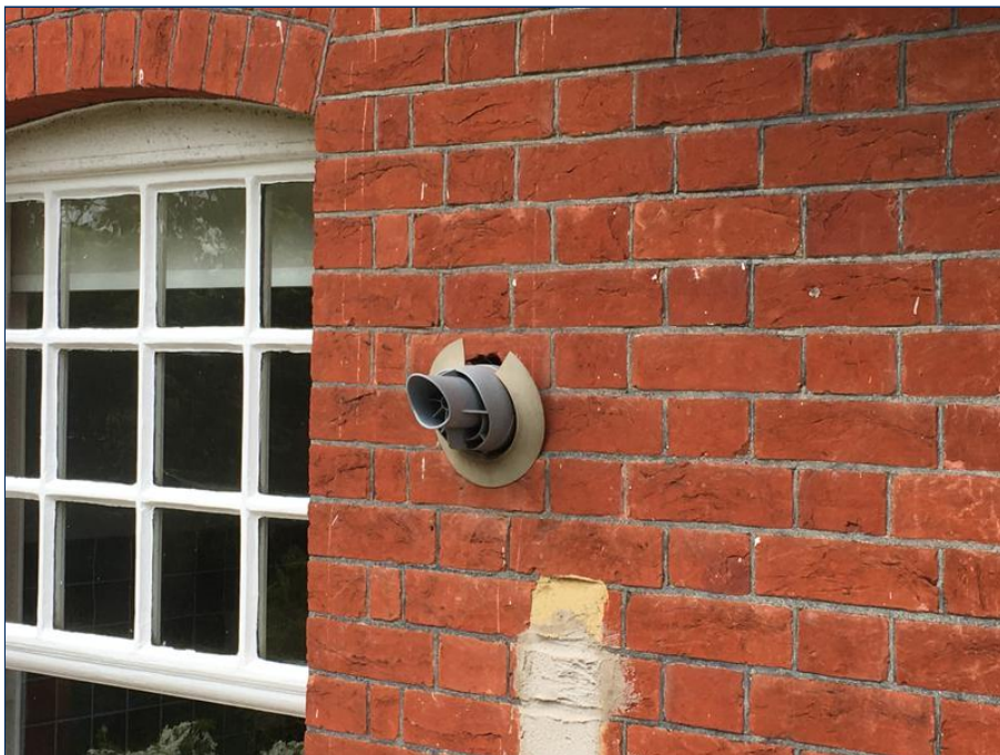
Photo 30 - Damaged collar
