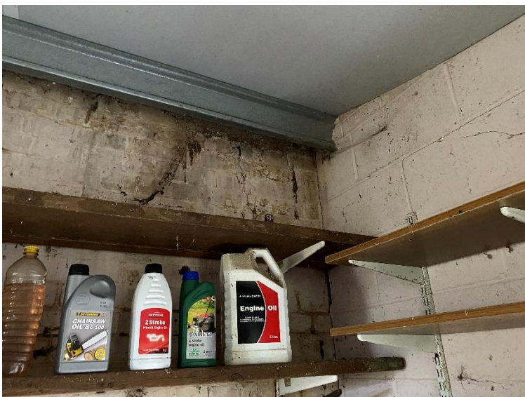
Evidence of leaks to the workshop.
