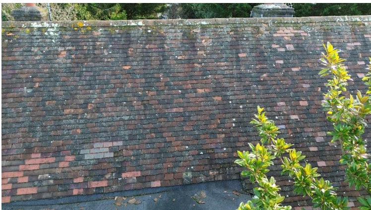
Widespread delamination to the east pitch of the south wing.
