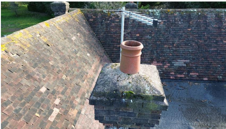
Cracked flaunching to the front stack.
