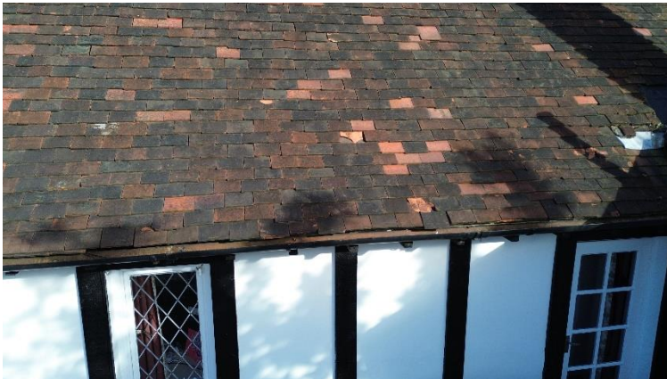
Delamination and broken tiles to the south pitch of the north wing.
