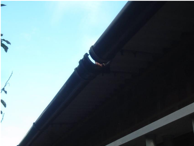
Defective gutters to the workshop.
